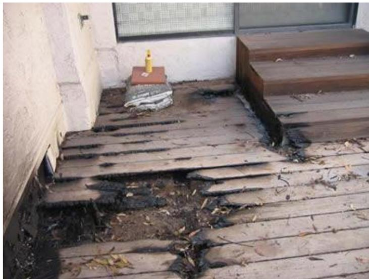
Spaces between deck planks can be landing spots for flammable embers
